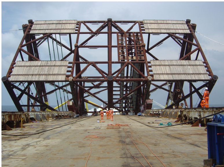
The 3000T Sumandak-B Jacket being launched from the CBL-102 Barge
